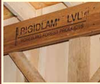
Glue LAM LVL header for increased snow loads and hurricane regions
